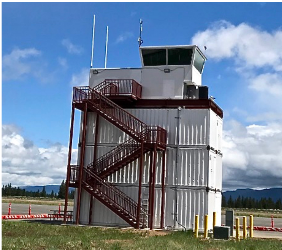
The Truckee airport traffic control tower looks like stacked cargo trailers. Photo/Carole Bernardi
