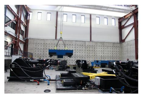
Three 27-ton, 14 x 14-foot table platens are lifted into place by the lab's 30-ton cranes as the lab crew continues installing equipment in the earthquake engineering facility at UNR. Photo/Mike Wolterbeek/UNR
