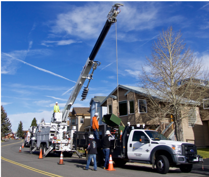
Crews maneuver the green transformer box into place. Photo/Kathryn Reed
