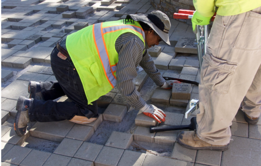
Workers on June 18 place pavers at Coyote Legacy Plaza. Photo/Kathryn Reed
