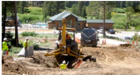
Kirkwood power house being built after the 2010 fire. Photo/Provided
