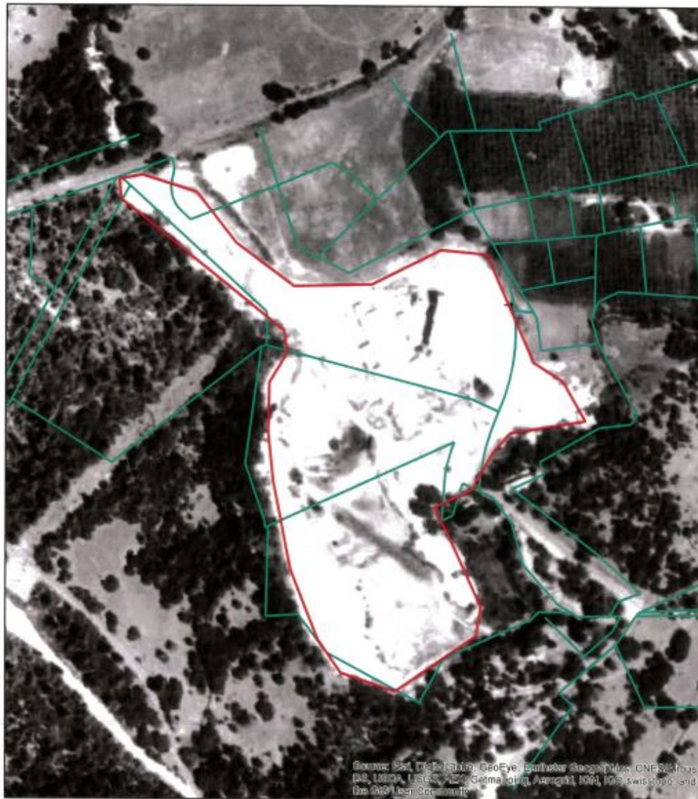
Figure 1 - Former Diamond Lime Plant Extent and Parcel Boundaries
