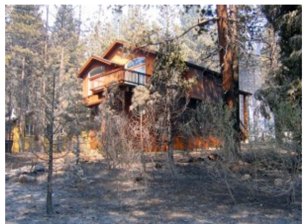
Proper defensible space
