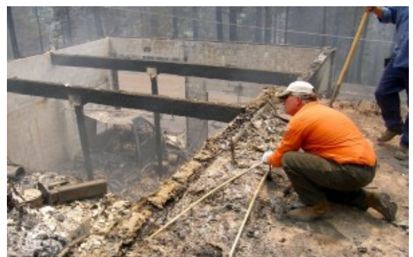
District crews crimp water supply lines in the burn area.
