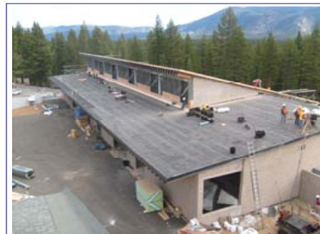
CTE Roof and South Wall
