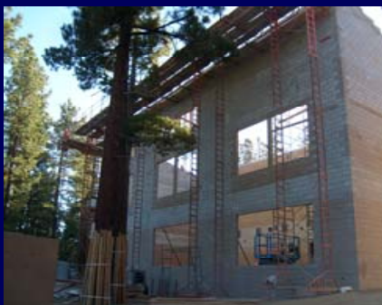
ORG-Exterior Masonry Walls-South West
