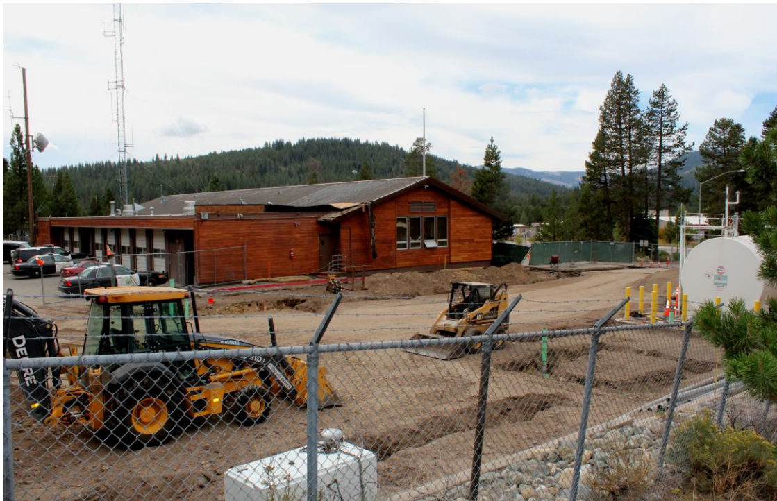
Figure 4.2. View of Proposed Vault Location (approximately between the two loaders)
