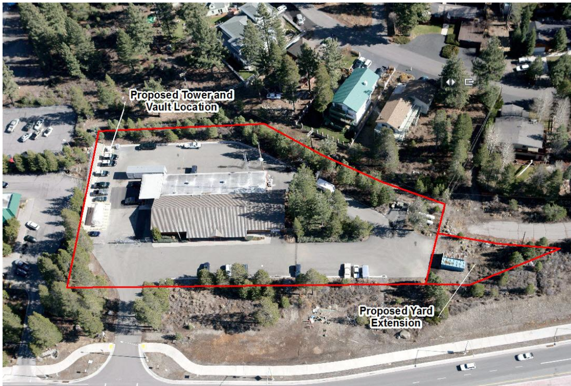
Figure 4.1. Oblique Aerial View of the Truckee Area Office Showing the Tower and Vault Construction Site and the \pm 0.09 -Acres to be Acquired
